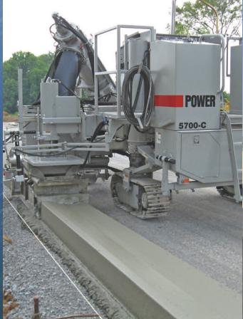
**CURB AND GUTTER** – The most productive machine in the world for parking lots, subdivisions and rehab curb. Turns 2' radius.
