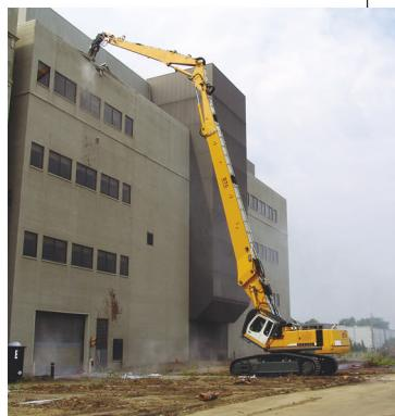
**Demolition excavator can reach 135 feet high with a 5,700-pound attachment to control high demolition.**
