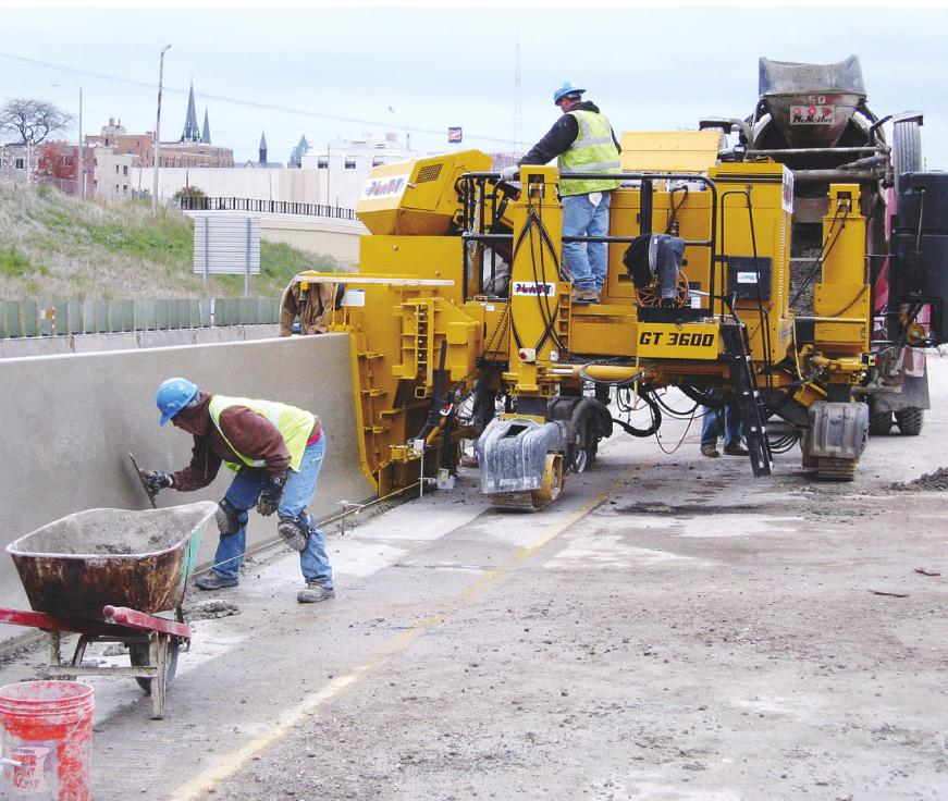
**GOMACO's GT-3600, GT-3400 and Commander III curb-and-gutter machines feature all-track steering, for quick setting to line. The operator simply crab-steers the machine sideways to get on the stringline, then flips the switch to forward-steer and takes off slipforming.**
