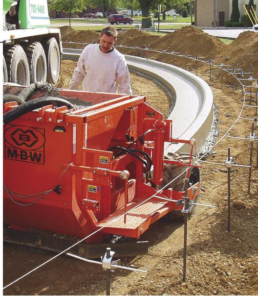
tor's starting to overload his hopper, then he can shut his conveyor down or have the truck stop pouring mud into the hopper.
