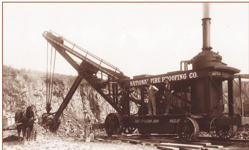
Usually mounted on traction wheels as shown in the illustration, “Little Giant” was used for lighter duties than the larger rail-mounted models.
